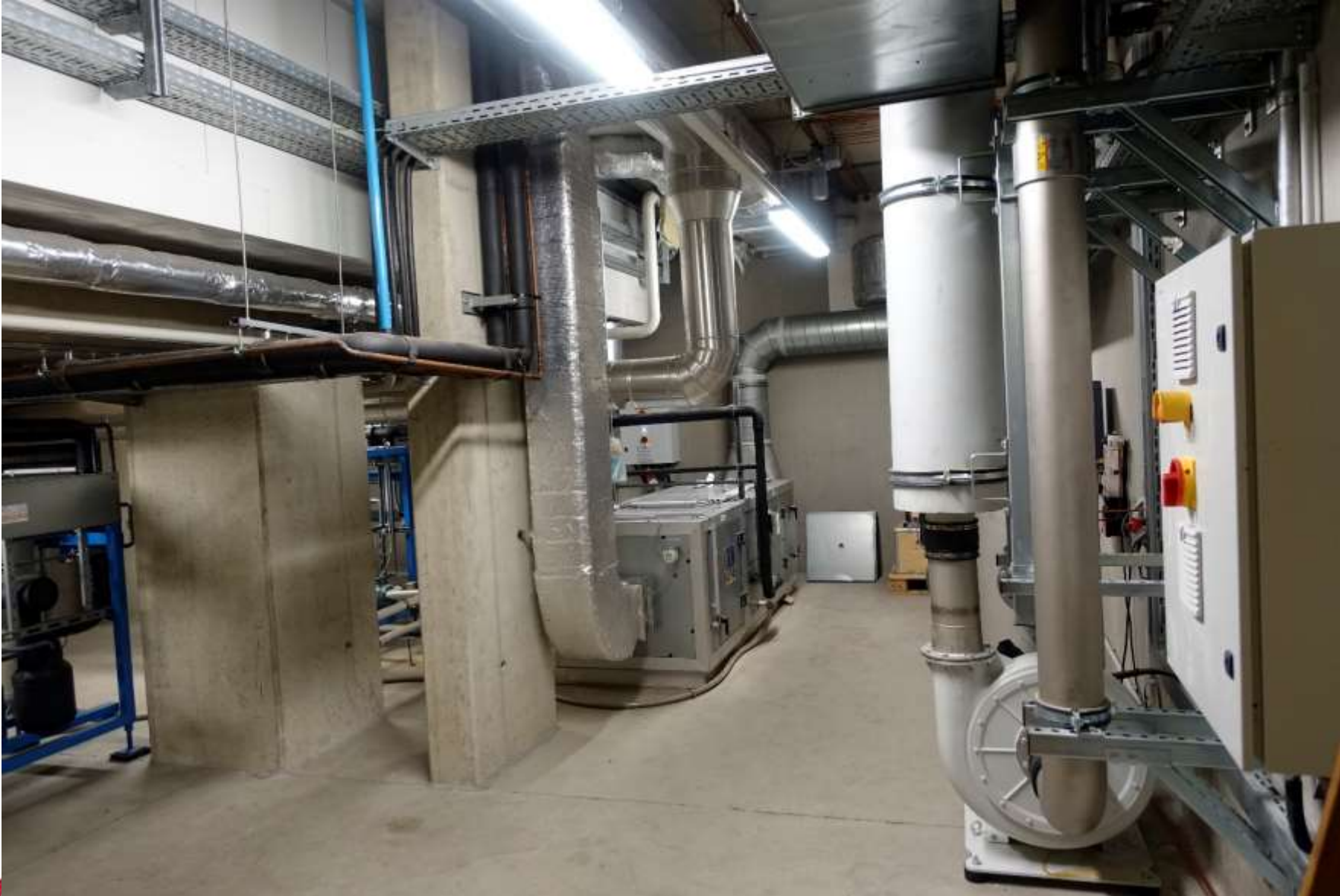
Air conditioning unit Blower
